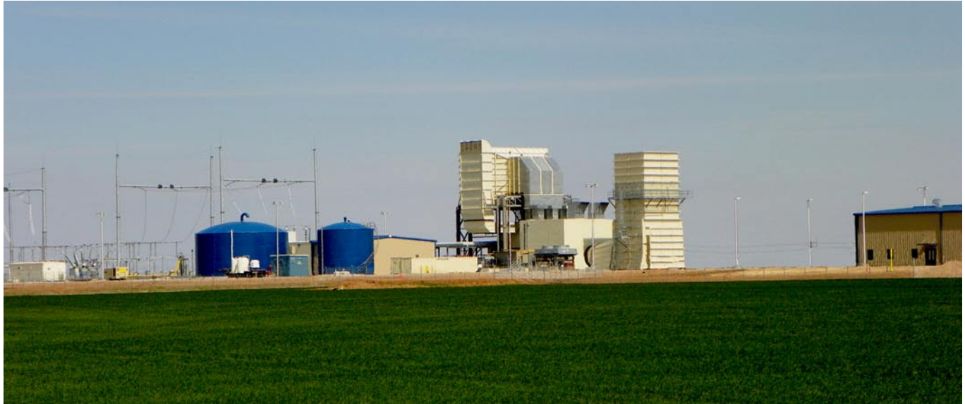
Charles D. Lamb Energy Center Ponca City, OK
