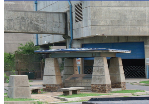
(Top) Kaw Hydroelectric Plant at Kaw Reservoir near Ponca City, Oklahoma (Left) Entrance to Kaw Hydroelectric Plant's powerhouse
